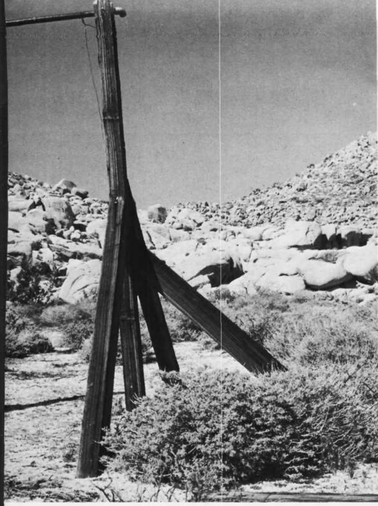
This frame structure was probably used as a hoist to unload heavy equipment at the upper camp of the San Diego and Arizona Railroad.
